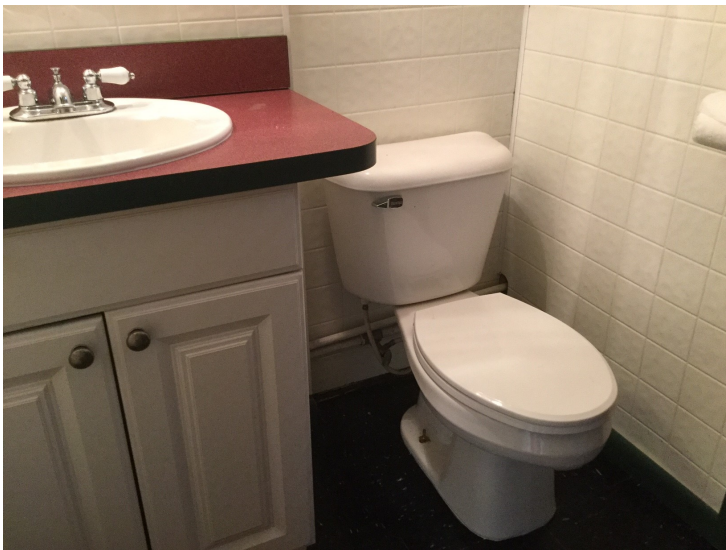
Above: New subfloor, new floor, fresh paint, and a good scrubbing of all surfaces have spruced up the artist's restroom after much-needed repairs were completed this summer.
